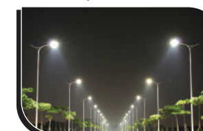
LED Street Lighting
