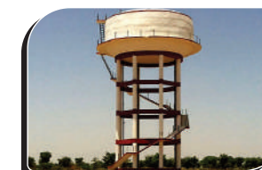
Dedicated Water Tank
