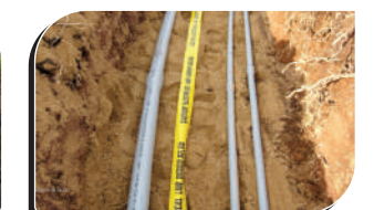
Underground Drainage, Electricity and Water pipeline
